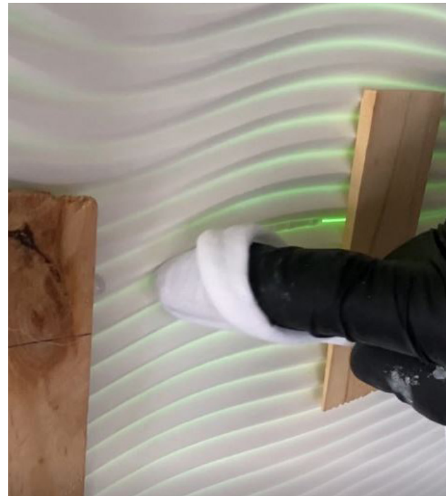
Wipe excess adhesive, wait 15-20 min to dry.
