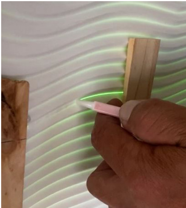
Add the adhesive topically between the seams.
