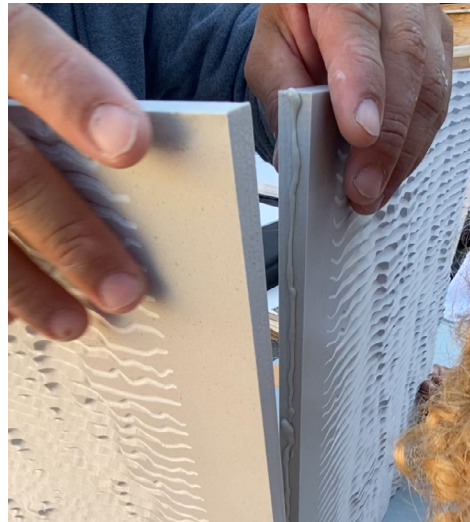
Add same colored corian adhesive to the butt joint seam.
