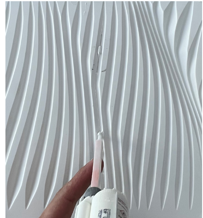
Step 3: Remove levelers and repeat in missing locations.
