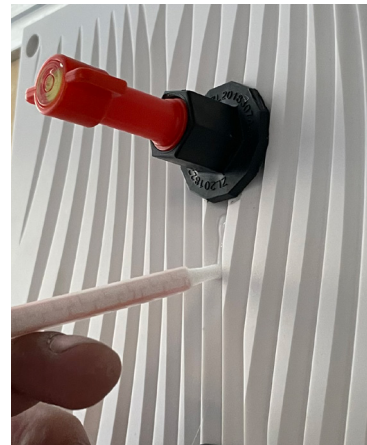
Step 3: Add a small bead of Corian to the seams. Corian Adhesive should ONLY be used topically.
