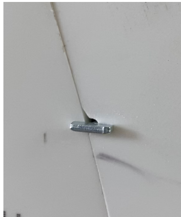
Step 2: Insert and twist the leveler so that the pin behind the surface is perpendicular to the seam. Hold and twist the leveler to tighten the seams together.
