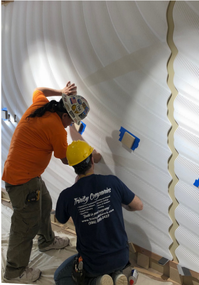
Leveling the faces using the stitching method
