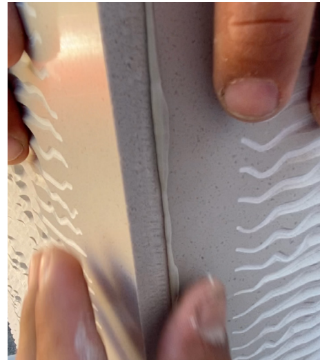
Squeeze butt joint together until adhesive beads out.
