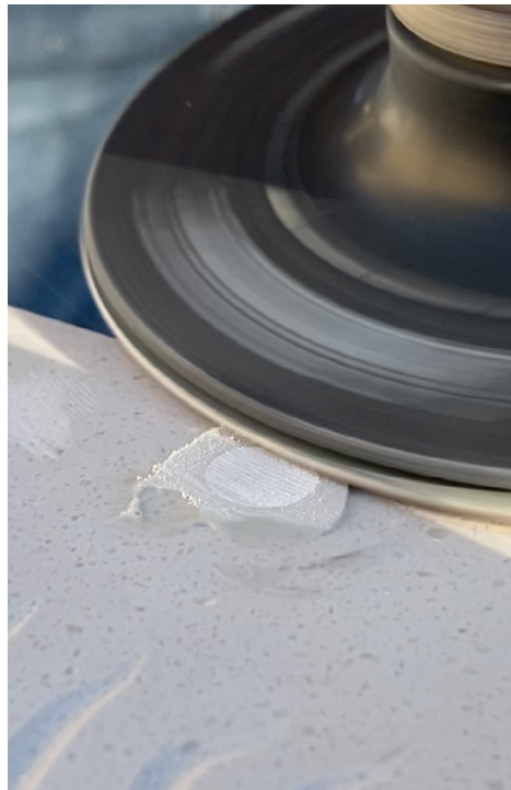
Step 2: Use grinder to shave down the exposed plug.
