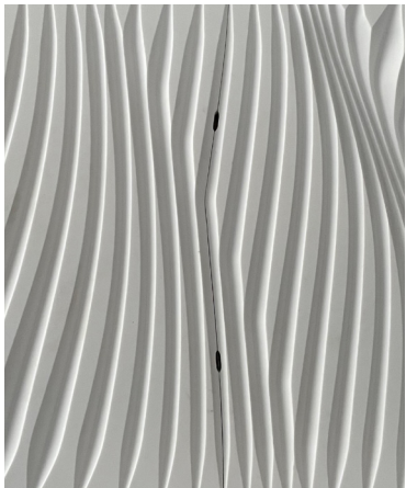
Step 1: Bring together two panels. Identify leveler slots.
