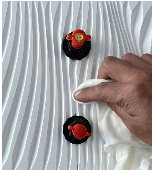
Step 2: With a clean rag, wipe excess adhesive, wait 15-20 min to dry.
