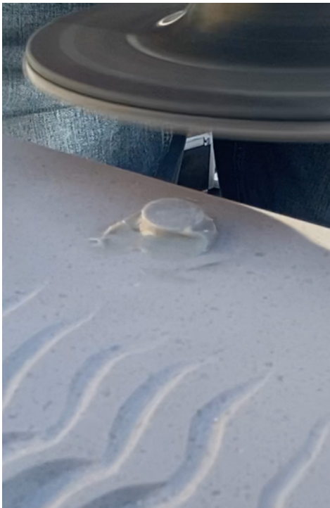
Step 1: Plug sticking out more than 1/32".
